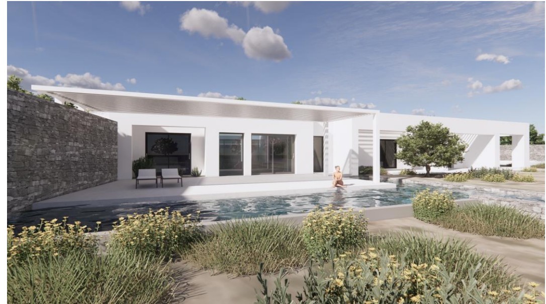
Exterior View of Villa B – pool & norther surrounding area
