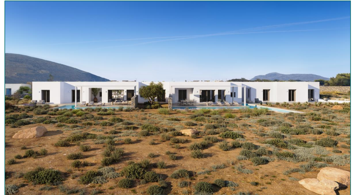
Exterior View of both Villas and surrounding area
