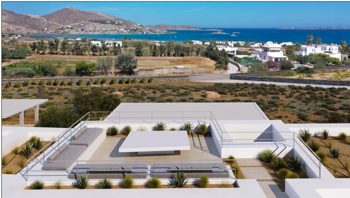
Accessible Roof area and View
